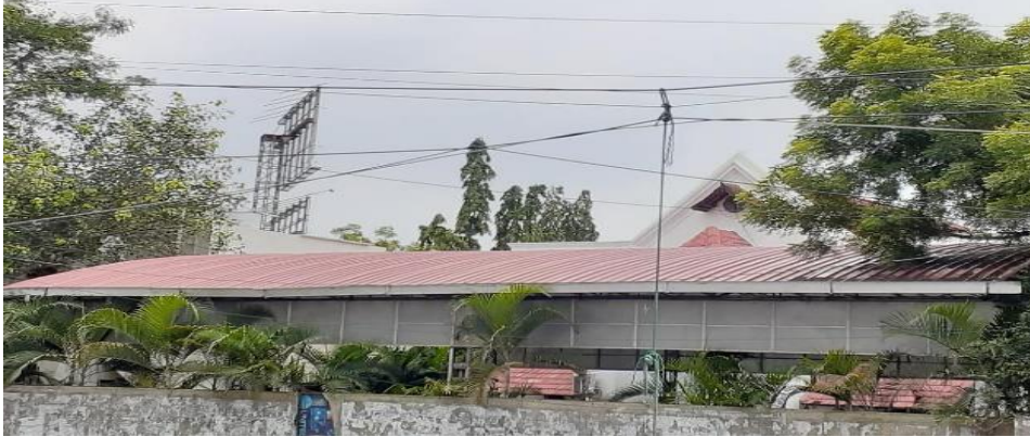
Repair and restoration of the Annex roof
